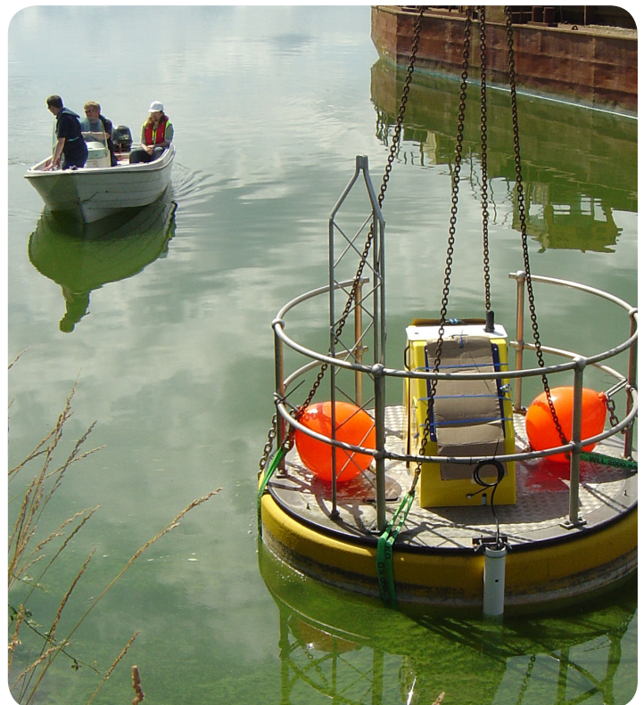
Preparing a floating water quality platform for installation.
